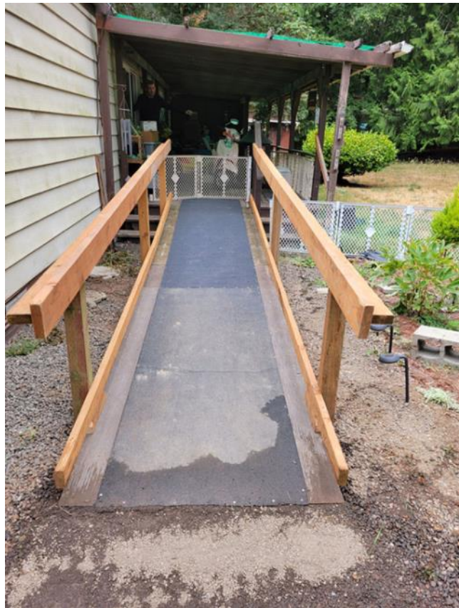
New Ramp – almost double in length and with added railings.
